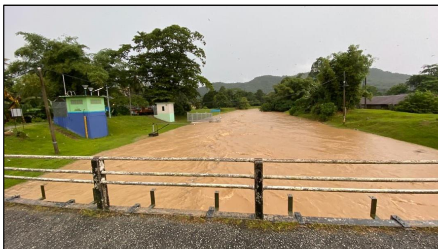
Figure 11. Bernam River at Tanjung Malim is turbid station during rainfall
