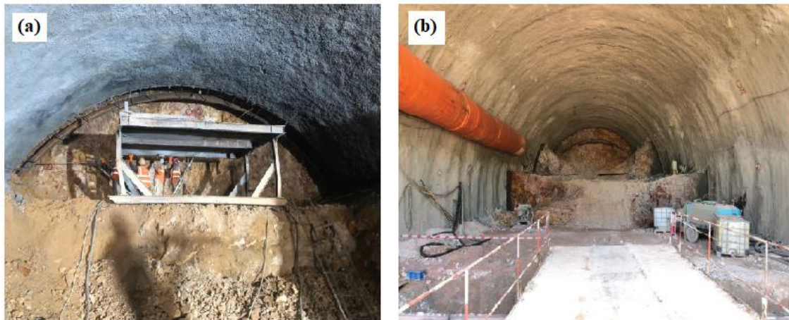
Figure 1.1 NATM excavation method use in ECRL project Malaysia
